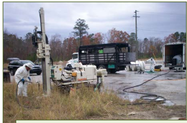
Integrated planning of bioremediation activities at Marine Corps Base Camp Lejeune enabled injections of emulsified vegetable oil and sodium lactate in four borings to be completed within only one week, which reduced field redeployment and associated fuel use.
