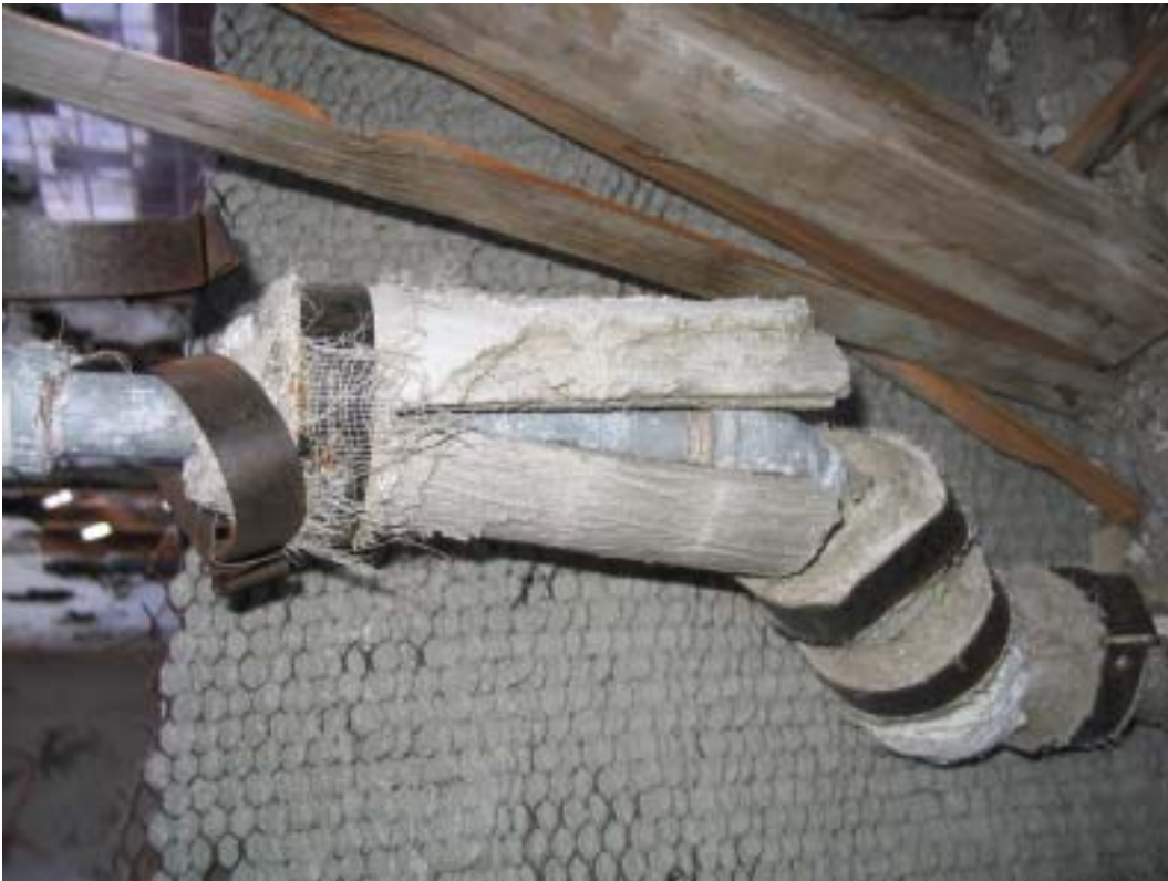
Photograph 6. Significantly damaged, friable ACM (pipe insulation).
