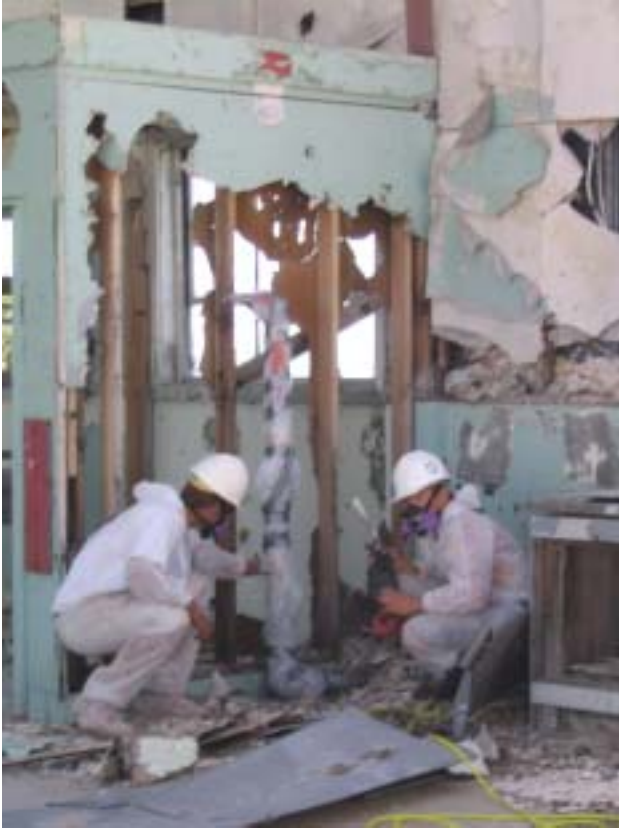
Photograph 19. Abatement workers prepare to remove a pipe with friable ACM.
