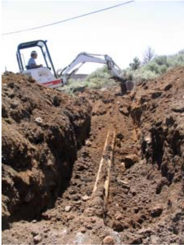
Photograph 29. ERRS excavates ACM steam line near the FAA facility.
