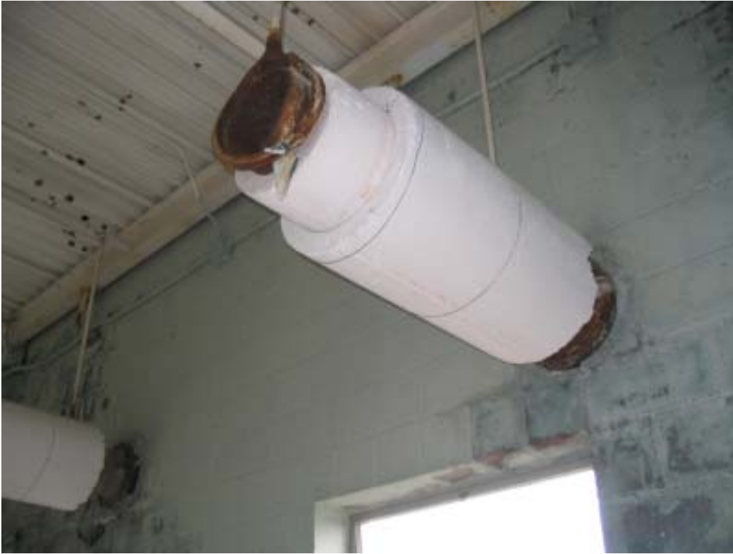
Photograph 7. Friable ACM (pipe insulation).
