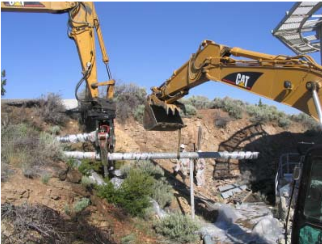
Photograph 28. Excavator with shears attachment prepares to cut ACM steam line.
