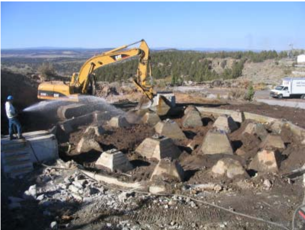
Photograph 34. ERRS backfills the foundation of Building 200.
