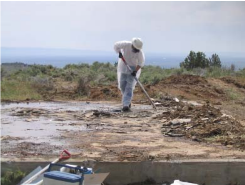
Photograph 20. Abatement worker removes ACM floor tile from concrete slab.
