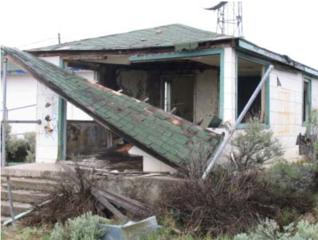
Photograph 10. Building 100, with collapsing roof.
