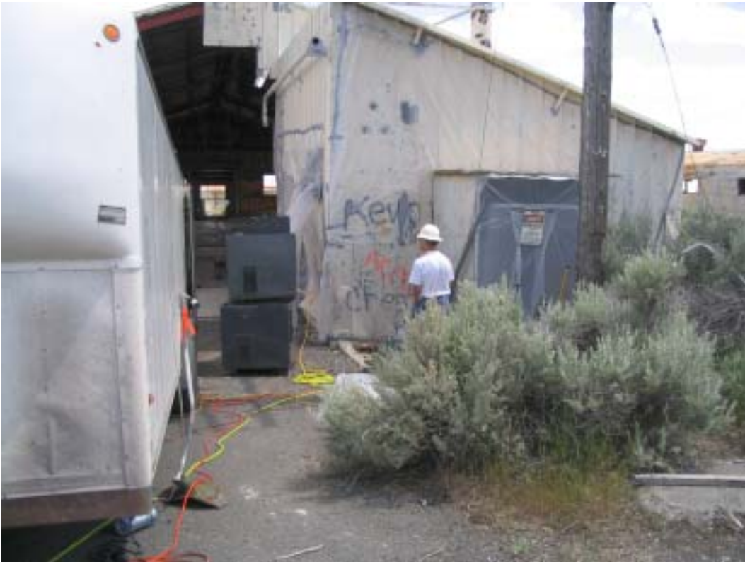
Photograph 18. Negative air enclosure for asbestos abatement at Building 155.
