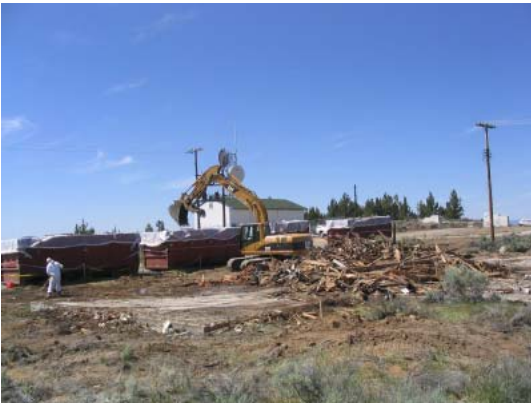
Photograph 36. ERRS loads ACM demolition debris into lined waste containers.
