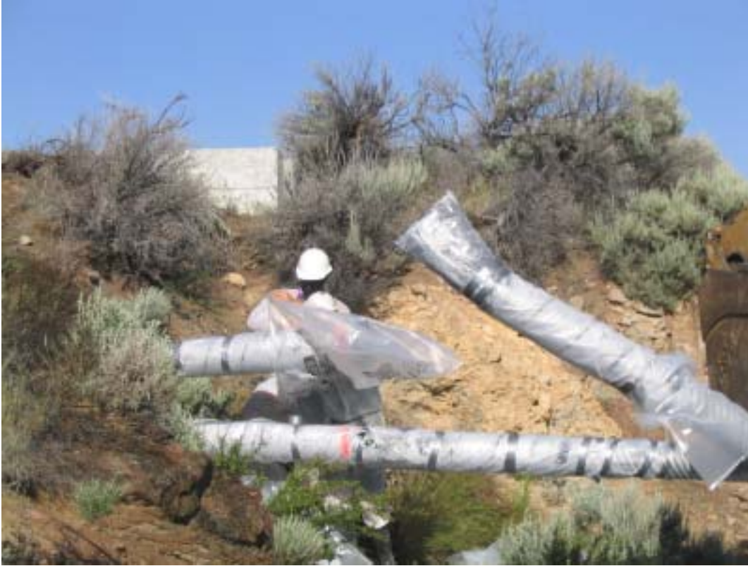
Photograph 27. Asbestos workers wrap the cut end of ACM steam line.
