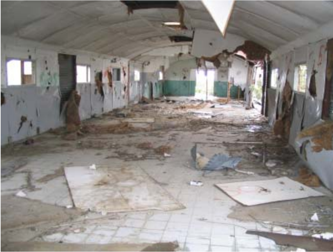
Photograph 11. Interior of Building 158, with damaged walls and ceiling.
