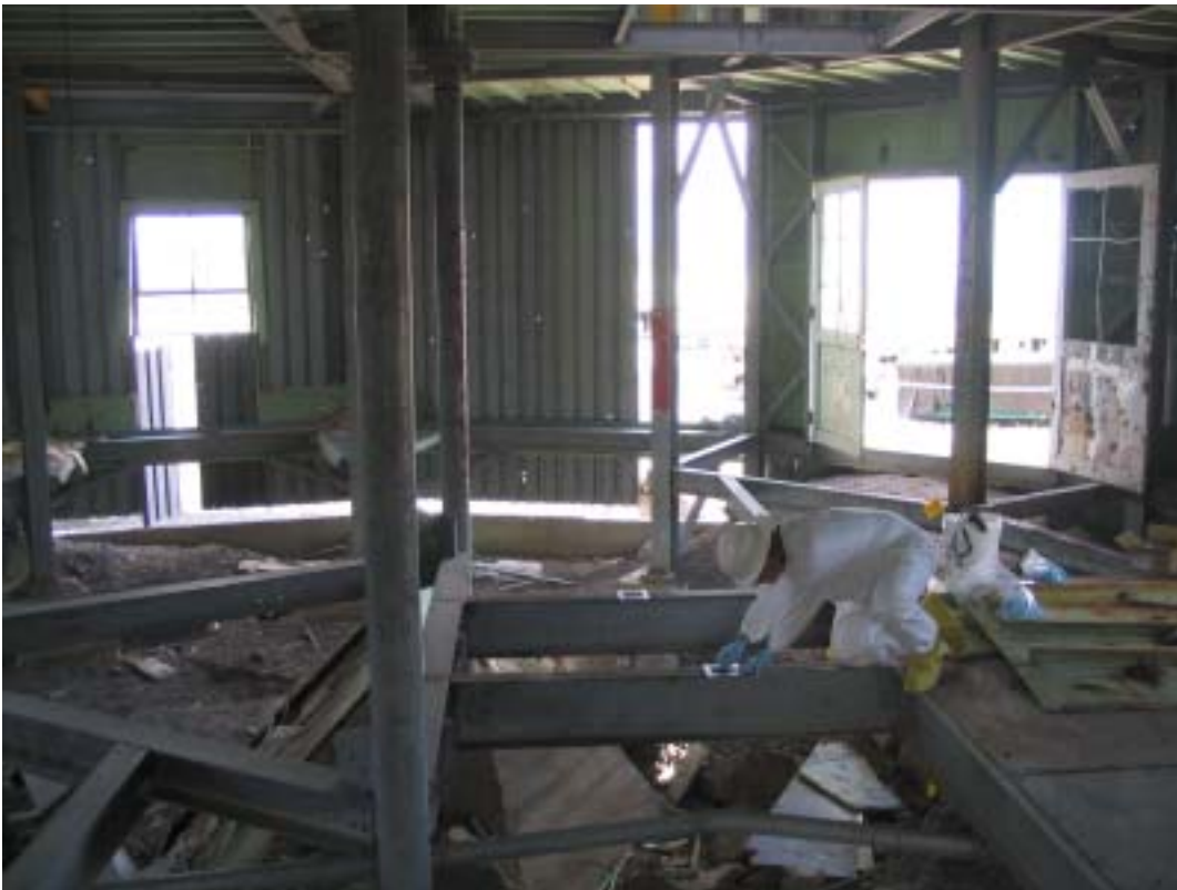
Photograph 14. START-2 collects wipe samples for PCBs inside Building 200 (radome).
