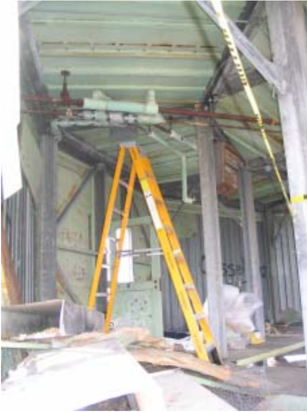
Photograph 17. Abatement worker prepares an ACM pipe run for removal.
