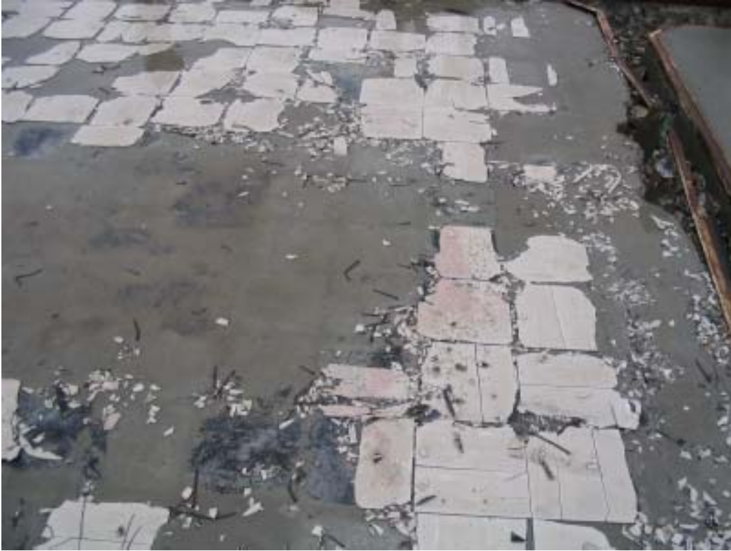
Photograph 9. Significantly damaged ACM floor tile.
