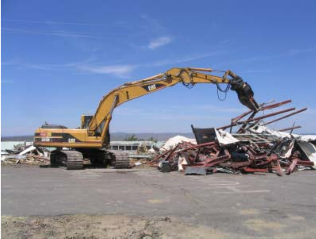
Photograph 37. ERRS separates scrap steel for recycling.
