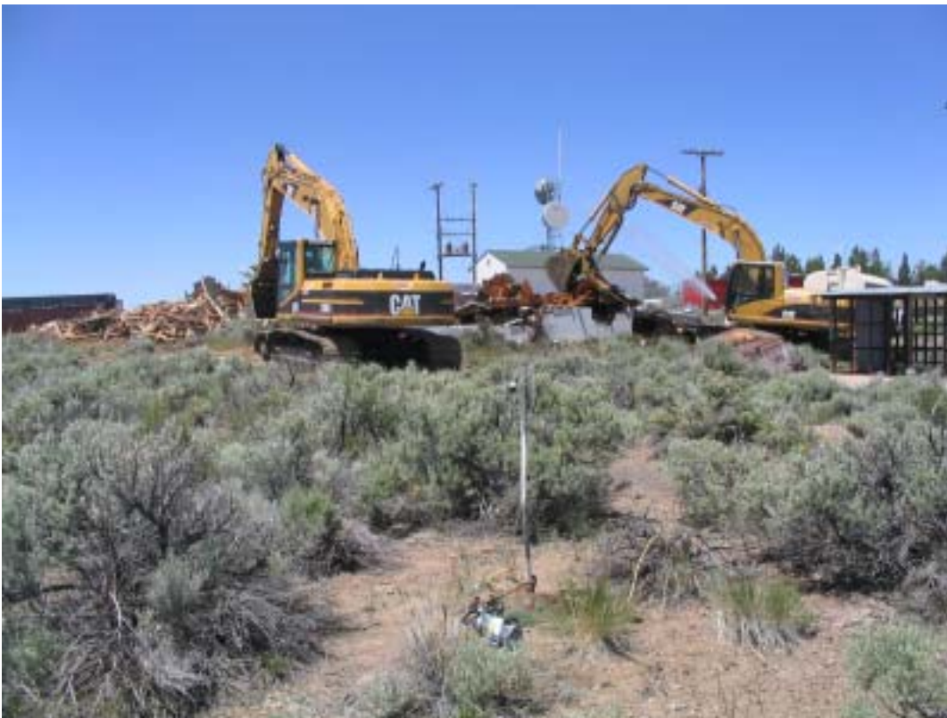
Photograph 32. Air sampling pump near demolition.
