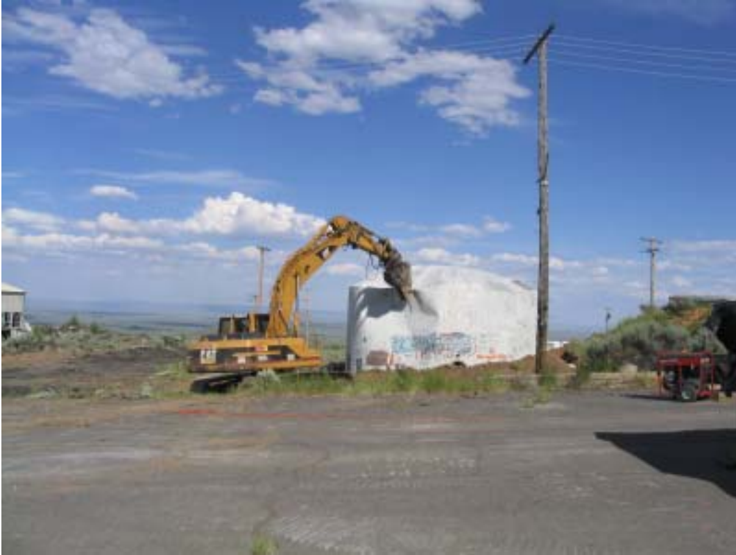
Photograph 23. Excavator with shears attachment demolishes Tank 804.
