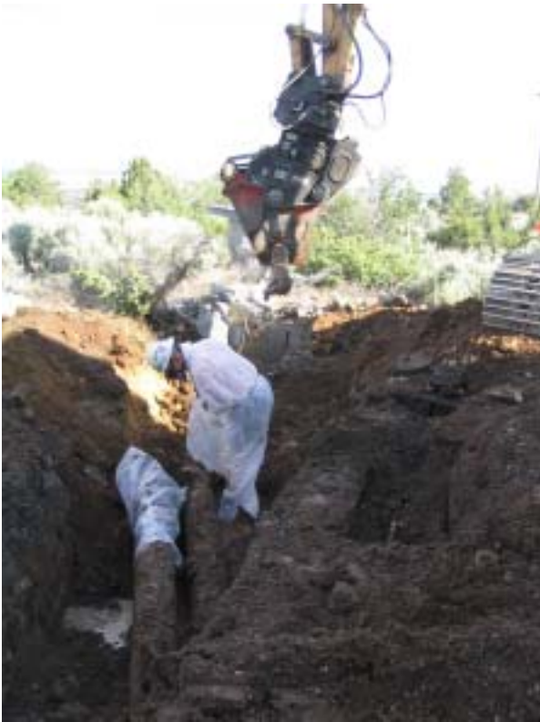
Photograph 30. Asbestos worker wraps excavated ACM steam line.
