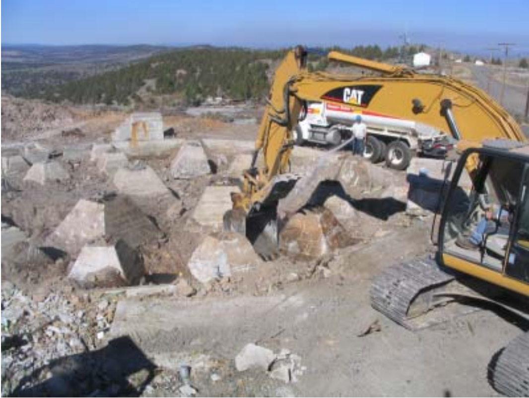
Photograph 33. ERRS excavates PCB-contaminated soil in foundation of Building 200.
