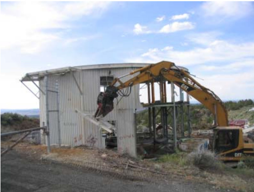
Photograph 24. Excavator with shears attachment demolishes Building 200 (radome).
