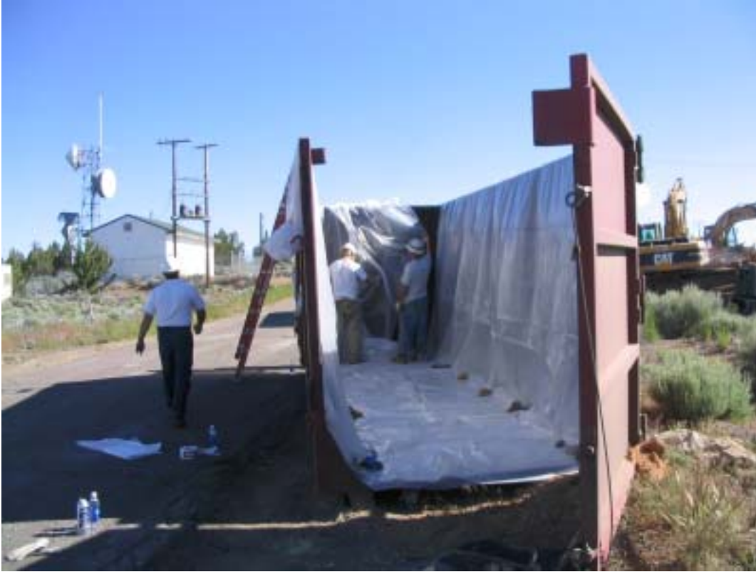
Photograph 35. ERRS lines an empty waste container for ACM demolition debris.
