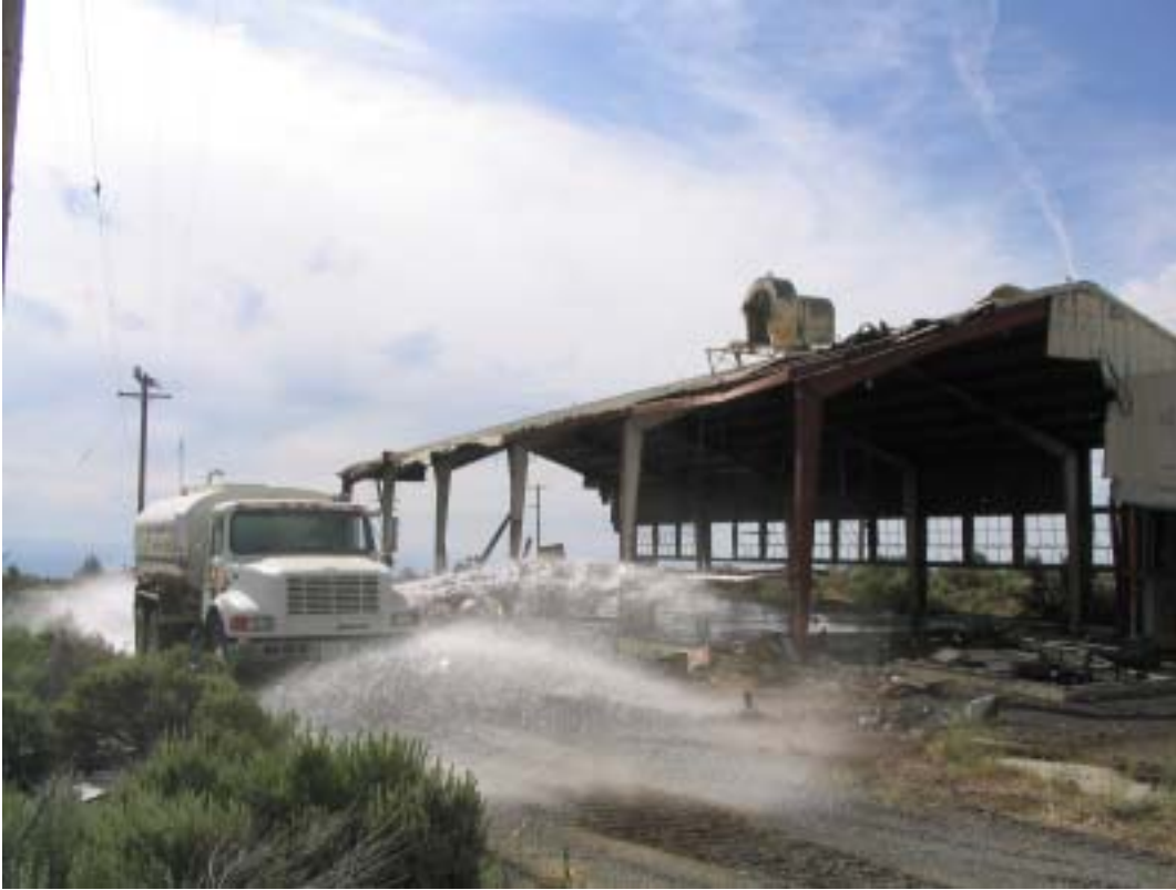
Photograph 25. ERRS water truck suppresses dust near Building 155.
