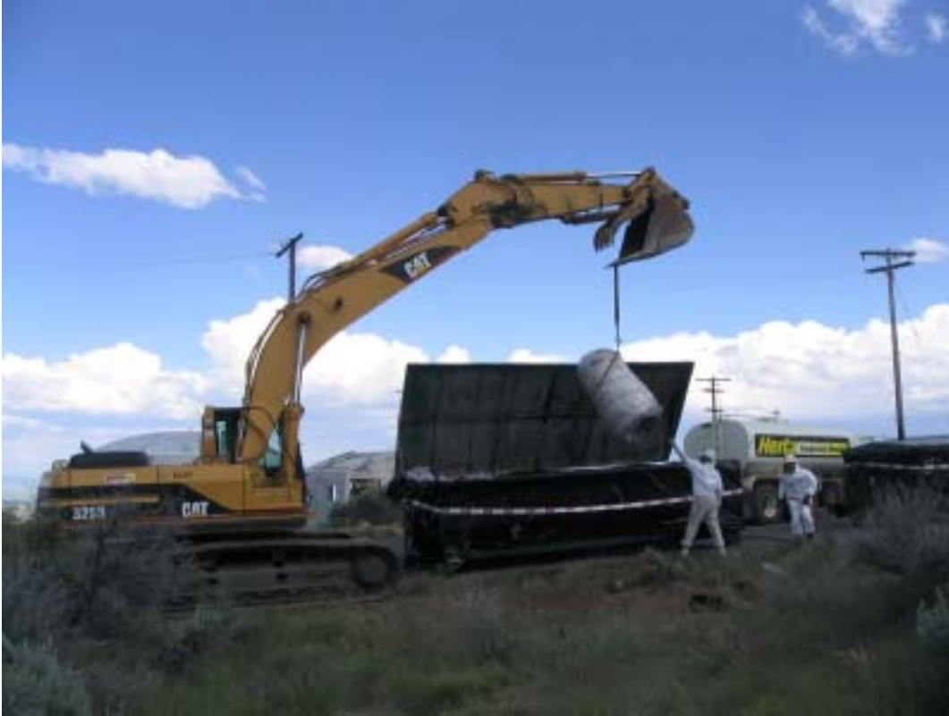
Photograph 21. ERRS loads a tank covered with friable ACM into waste container.
