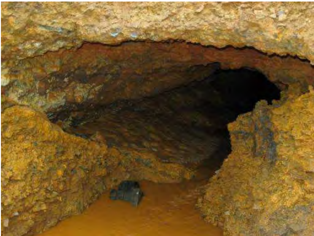
PHOTO 40 9-29-2011 Left rib of adit. Abundant collapse/fines/yellow boy material.
