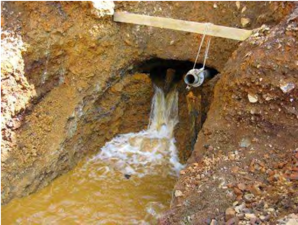
PHOTO 39 9-29-2011 AMD water flowing from adit.
