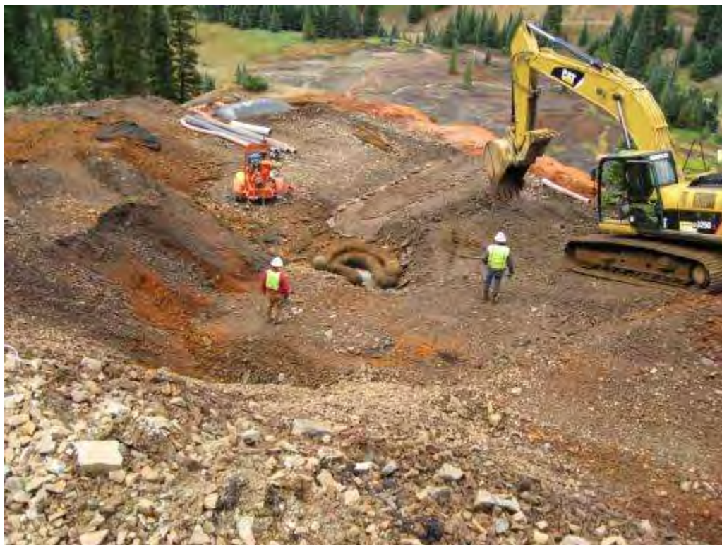
PHOTO 32 9-15-2011 View of operations on top of dump. Collapsed portal behind nearest workman's back out of view in foreground, AMD water flowing through temporary rock dam (nearest workman standing on) to sump where Koir-Logs® are located, under-piped to geotextile filter bag in background (behind stacked piping) where water is filtered prior to release to the south ditch out of view. AMD water flows through stressed vegetation zone in photo background to Cement Creek.
