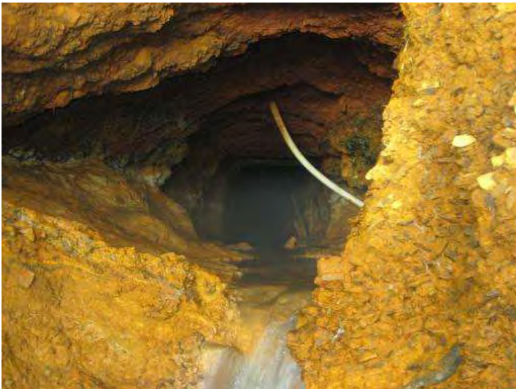
PHOTO 44 10-11-2011 View into adit from portal. Sediment material on floor in photo foreground is 2 feet thick, approximately 4 feet of open space to adit back. AMD water draining down center. PVC monitoring well pipe is visible in adit. Note timber set visible behind PVC well.
