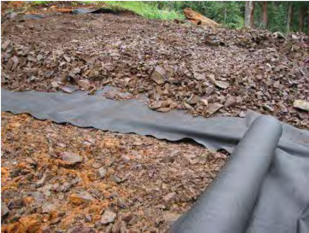
PHOTO 17 8-31-2011 Geotextile fabric placed between layers of talus material on mine dump.
