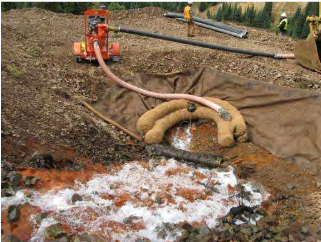
PHOTO 22 9-10-2011 Koir-Logs®, filter barrier, and pump at sump below the adit outflow. Twelve-inch PVC pipe under Koir-Logs® directs water to south ditch when not being pumped to manifolded filter bag apparatus at toe of dump. Pipe can be plugged with stopper, stored on Koir-Log® in photo center.
