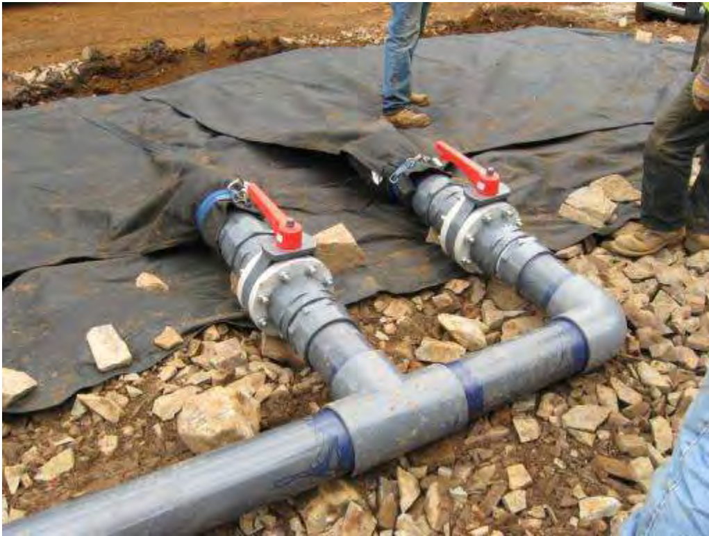
PHOTO 21 9-10-2011 Valve and filter bag manifold apparatus. Unused bags.
