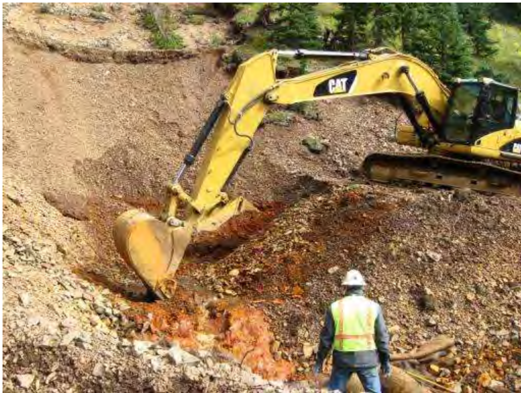
PHOTO 31 9-13-2011 Excavation activities at collapsed portal.
