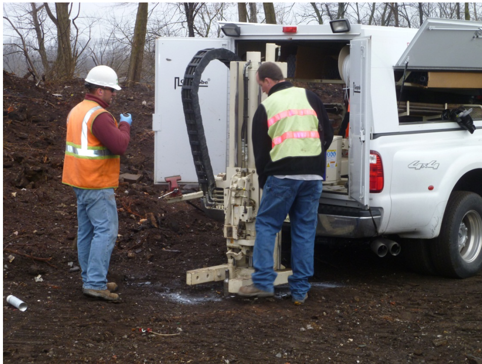
Photograph No.: 6 Photographer: Santino Nardulli Orientation: Looking Northeast TDD Number: TO-01-12-10-1012 Contract: EP-S5-10-10, OTIE Date: 12/03/12 Site Name & Location: Dixon Road Site, Kokomo, Howard County, Indiana Subject: View of subcontractor Ark Engineering obtaining soil boring.
