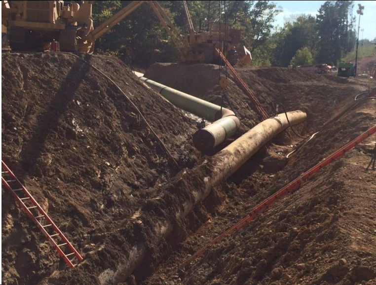
By-pass tie-in line where it will be connected to main line.
