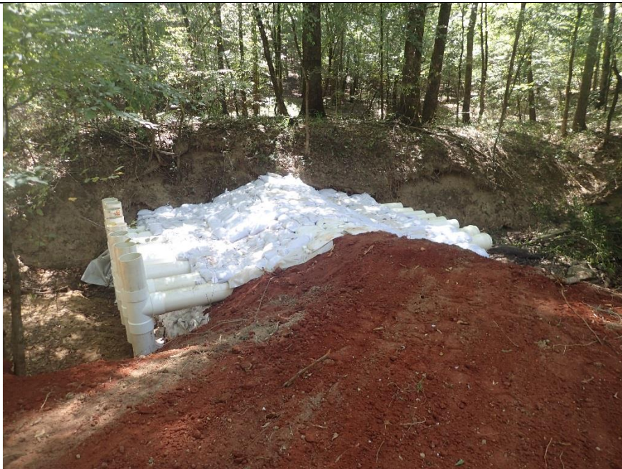
Completed underflow dam in Peel Creek, approximately 200 feet southeast of the Cahaba River.
