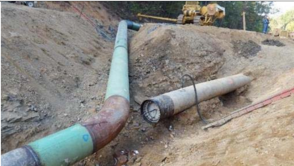
Operations completed the by-pass tie-in.
