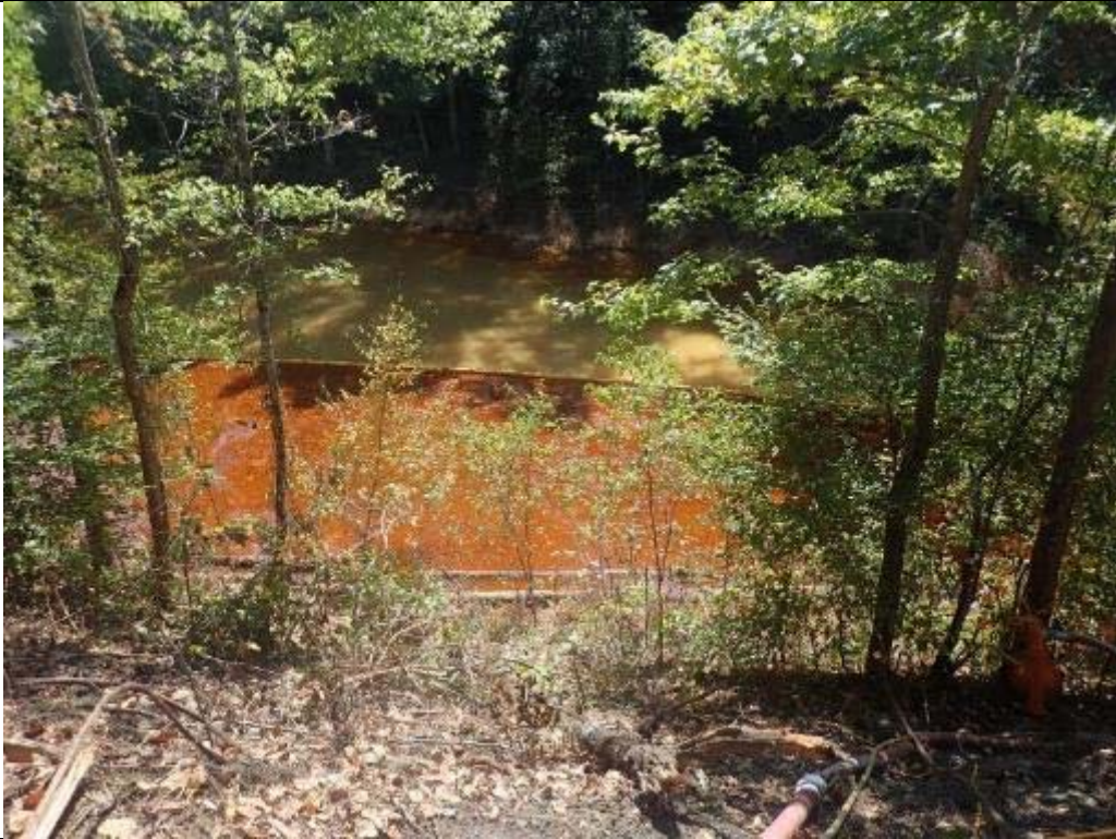
Crews corralled product on Pond 2 at recovery point 2b to better remove it via skimmers.
