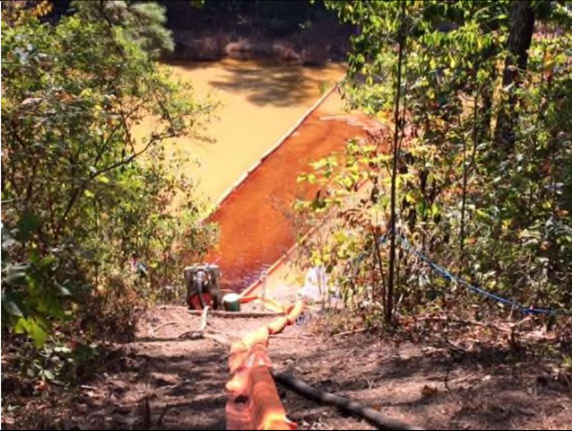
Crews corralled product on Pond 2 at recovery point 2a to better remove it via ray skimmers.
