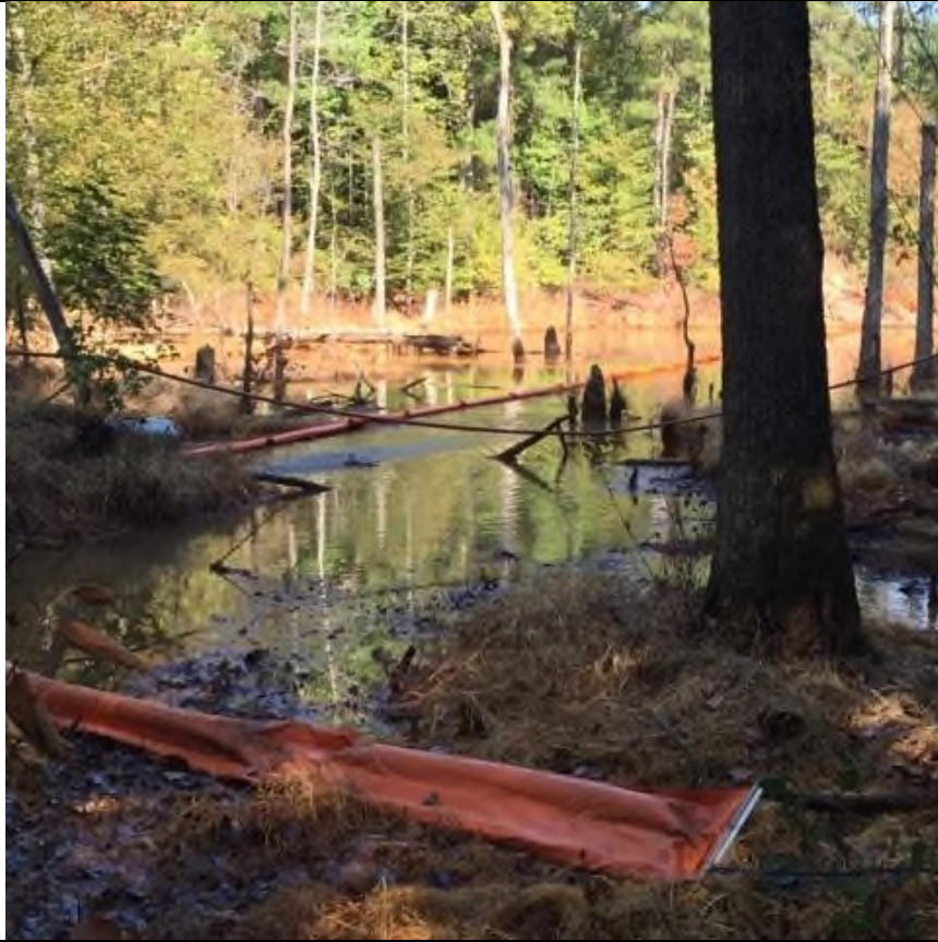
Containment boom deployed in Pond 2 at the mouth of the ravine.
