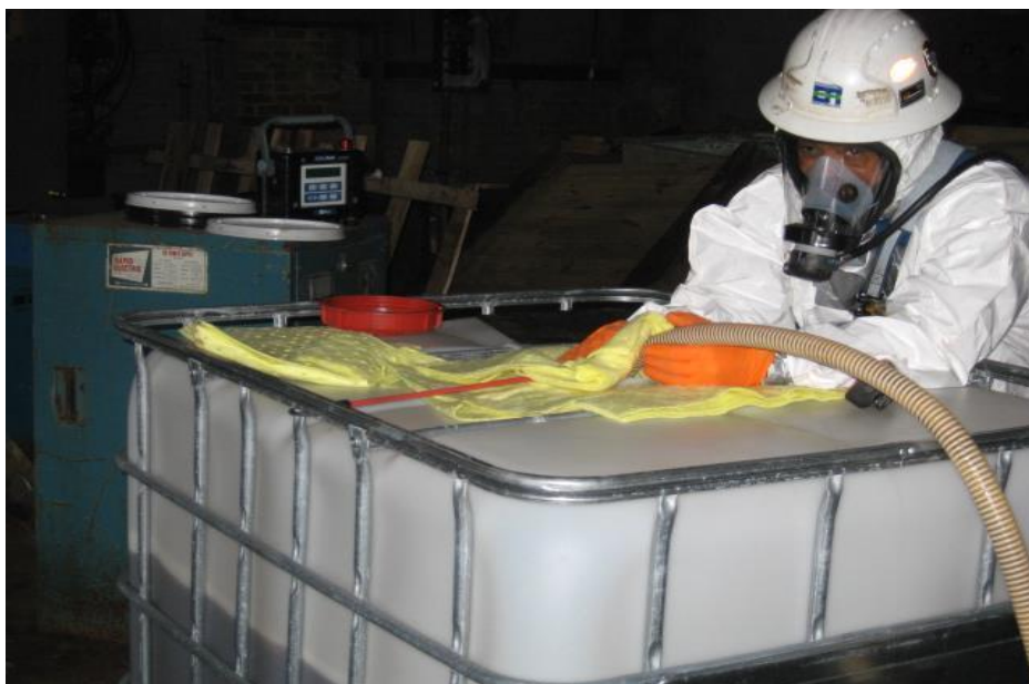
PHOTO 9: Bulking of compatible hazardous materials for disposal with area monitoring device in the background.
