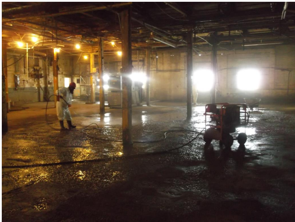
PHOTO 15: Pressure washing the floor of the building after hazardous materials and electroplating lines and vats had been removed.
