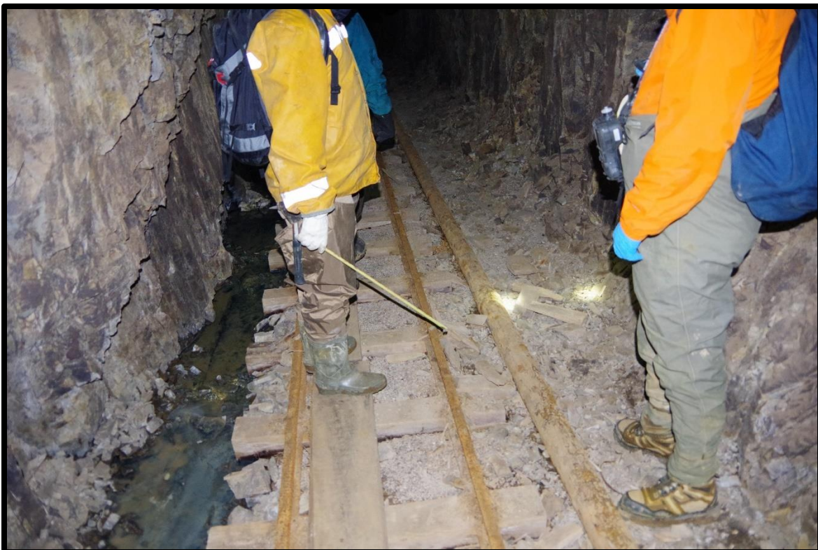
Photo 8: Typical rail, ditch, and invert in Commodore 5 Cross Cut
