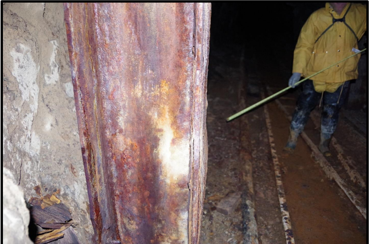
Photo 34: Close up of Archimedes Raise steel posts; Note corrosion and delamination
