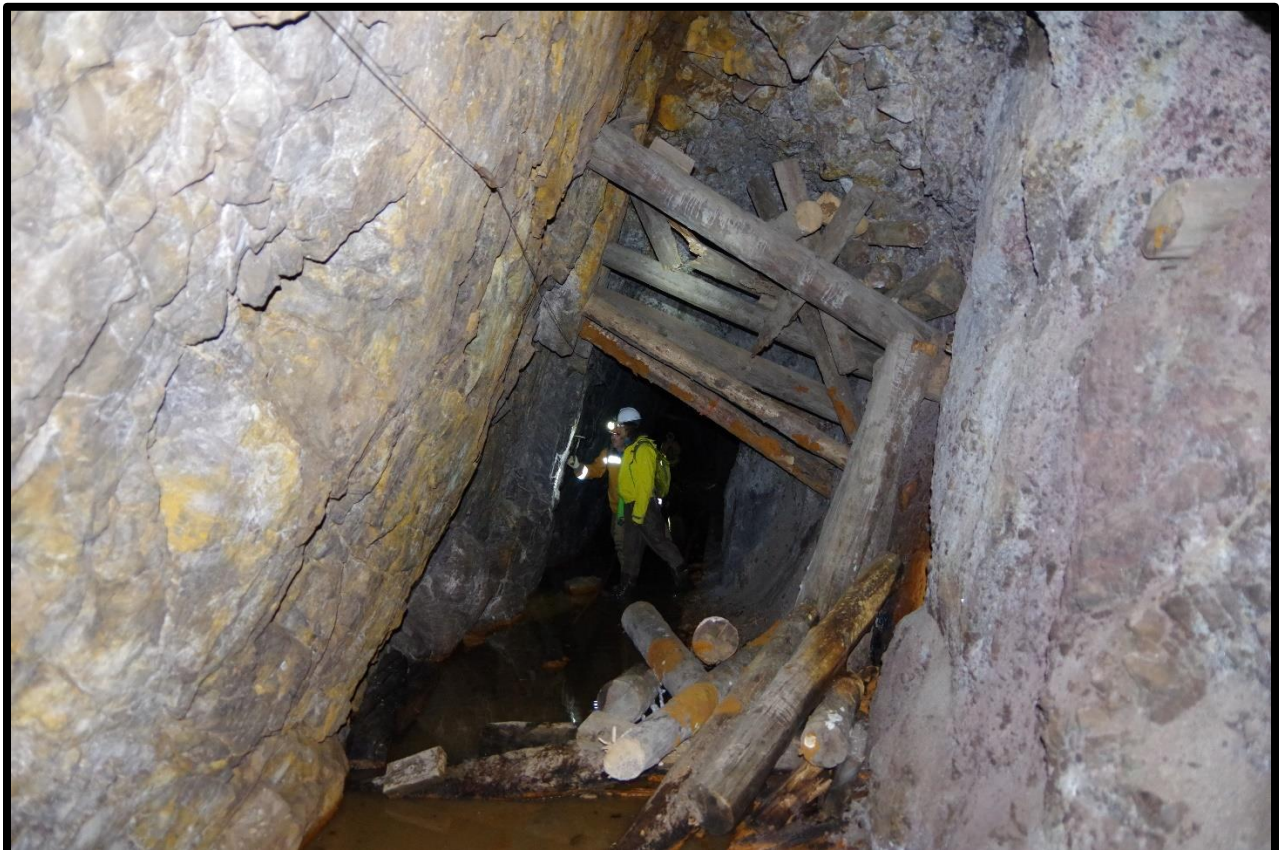
Photo 40: Failed timber stulls near 32+80
