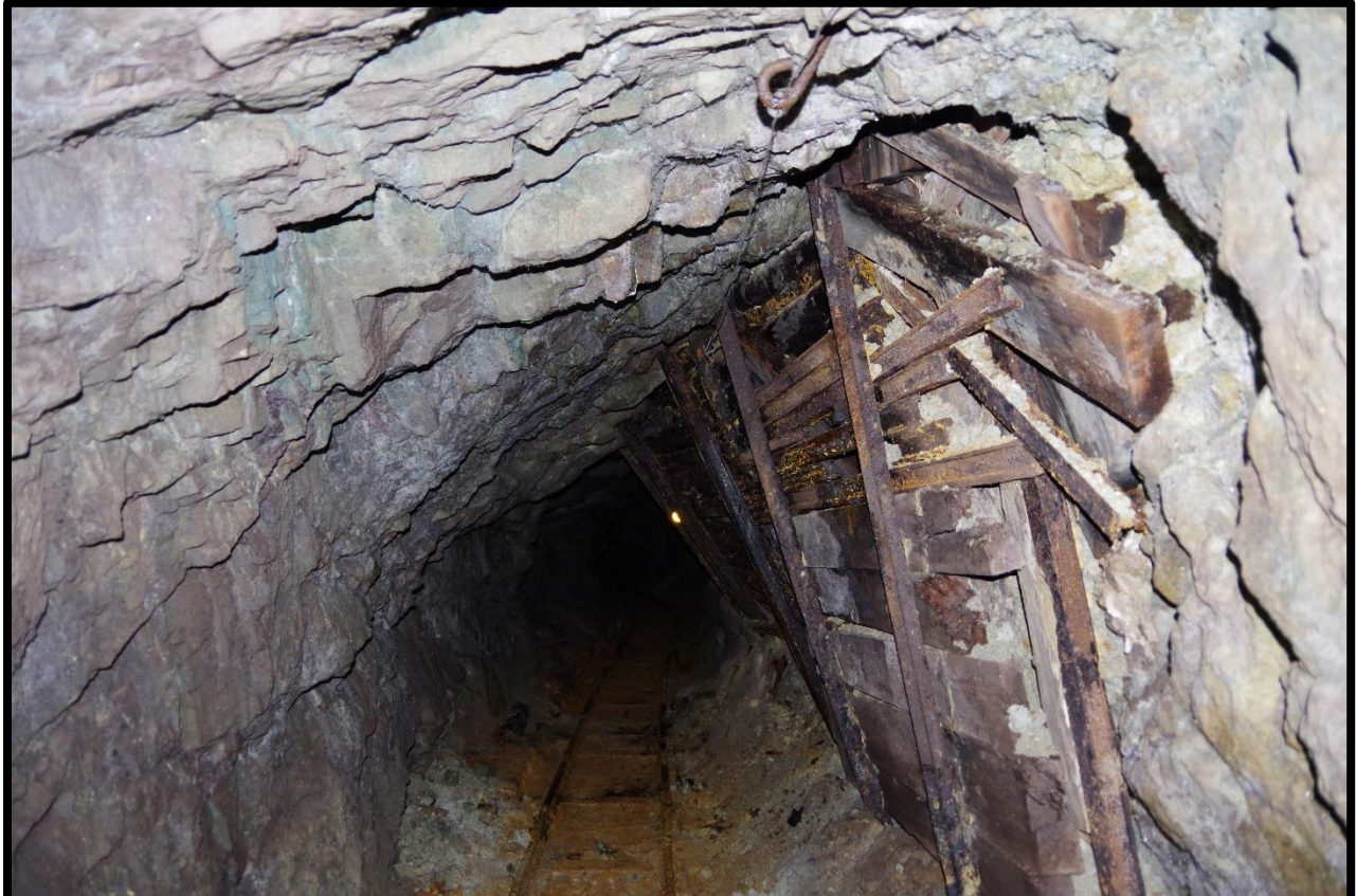
Photo 58: Area of clay gouge in left rib near 47+10 looking outby; Note timber lagging
