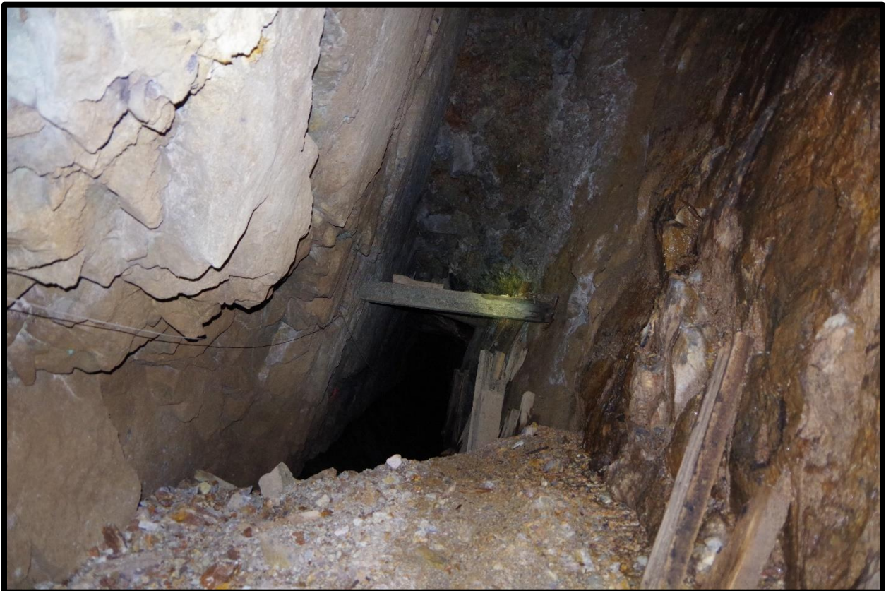
Photo 41: Debris pile at very active 44 Raise 36+82
