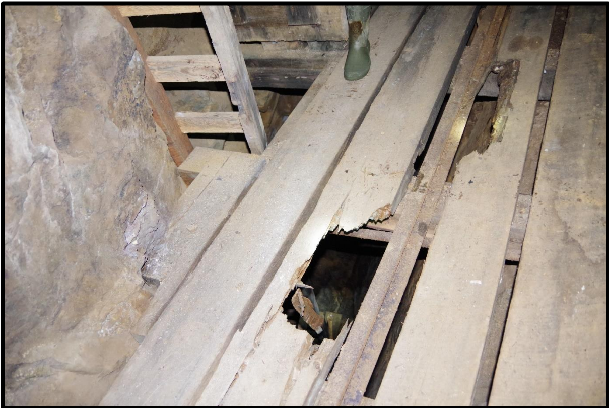
Photo 17: Daylight Winze with rotten wood cover
