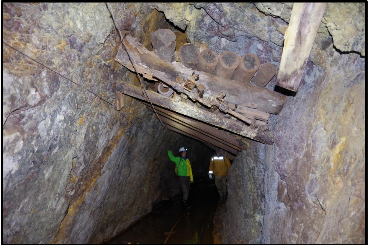
Photo 39: Steel pipe stulls near 32+20; Note pipe cribbing
