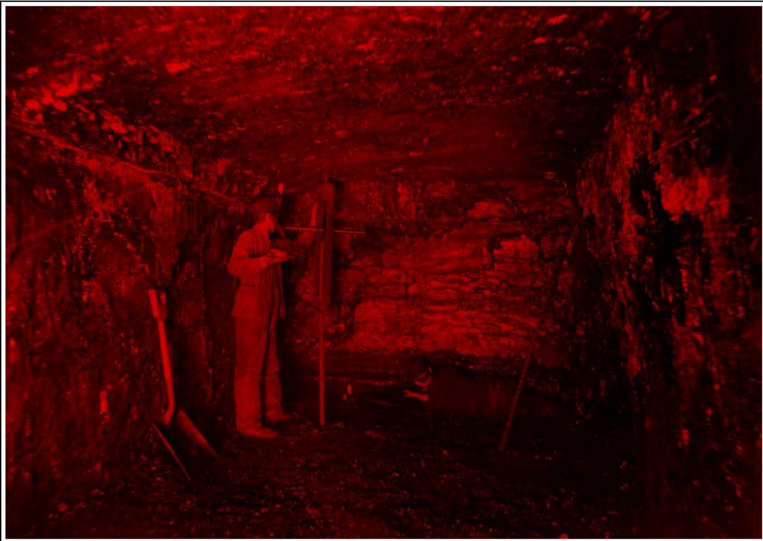
TWO MINERS PREPARING TO BLAST THE COAL. THE MAN STANDING IS DRILLING THE FACE IN ORDER TO PLACE HIS POWDER, THE MAN LAYING DOWN IS UNDERCUTTING THE COAL TO AVOID A WINDY SHOT AND ALLOW THE COAL TO DROP TO THE MINE FLOOR IN CHUNKS READY FOR LOADING. NOTE THE TYPE AND LOCATION OF THE MINER'S OIL LAMPS. UNION PACIFIC COAL COMPANY. (UNDATED) (WYOMING STATE ARCHIVES, DEPARTMENT OF STATE PARKS AND CULTURAL RESOURCES)
