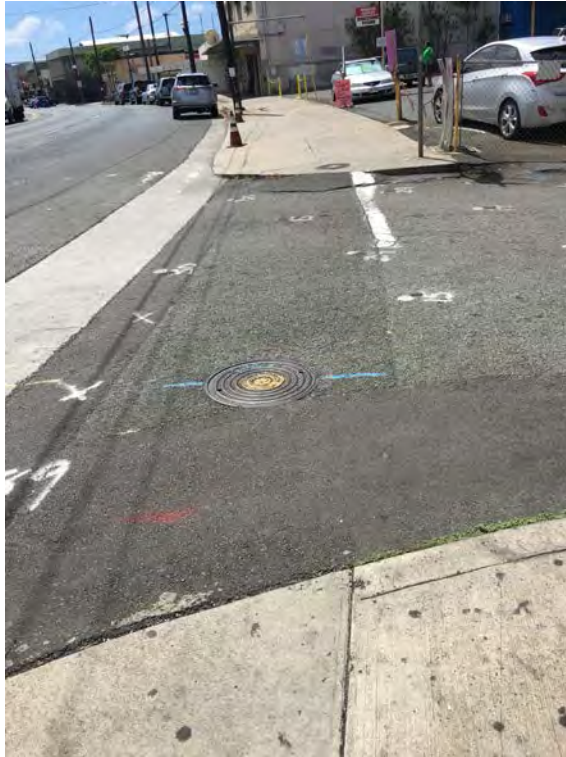
Photo 1 : Corner of Factory Street and N. King Street looking (view towards Diamond Head). Red marks show locations of electrical lines, blue marks locations of water lines.
