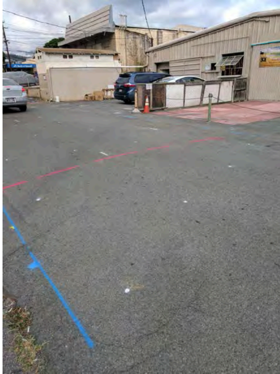
Photo 4 : Factory Street viewed towards east/northeast. Water lines (blue) are marked on the Ewa side (left) and an electrical line (red) is marked crossing Factory Street.
