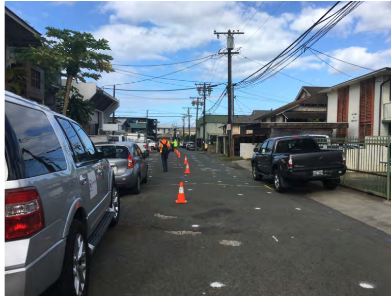
Photo 2 : Factory Street viewed towards southwest. Water lines (blue) are marked on the Ewa side (right) and crossing Factory Street. The yellow line crossing the street indicates the presence of a gas, petroleum, or steam line.
