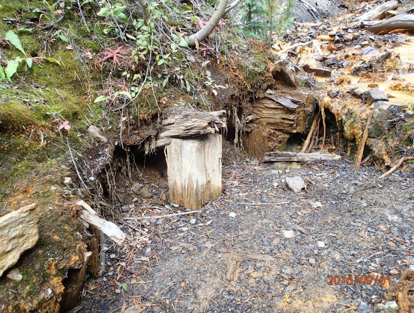
Drainage emerging six feet above cap timbers indicating that the adit is flooded
