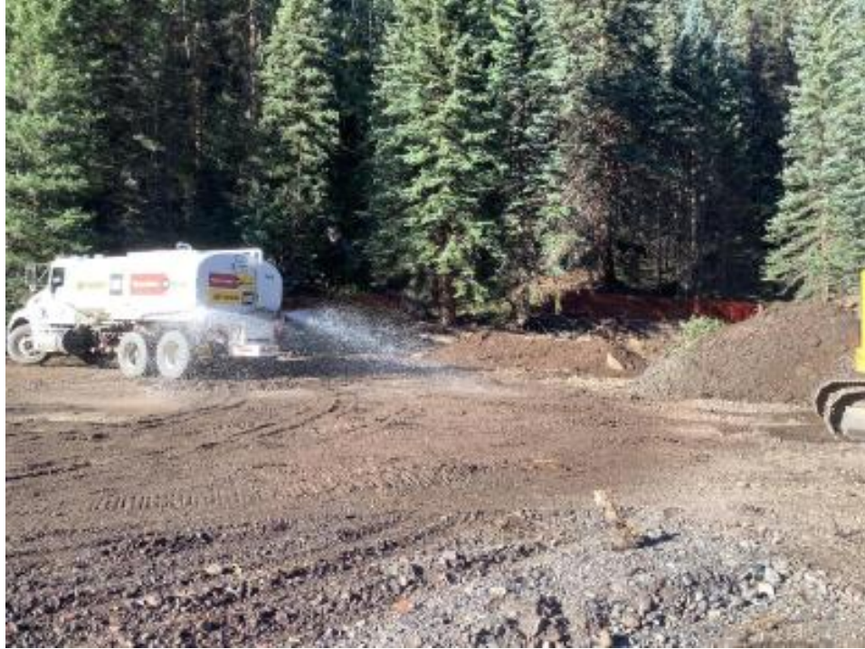
Water truck sprays down work area as excavator removes tailings in western boundary of ST2.
