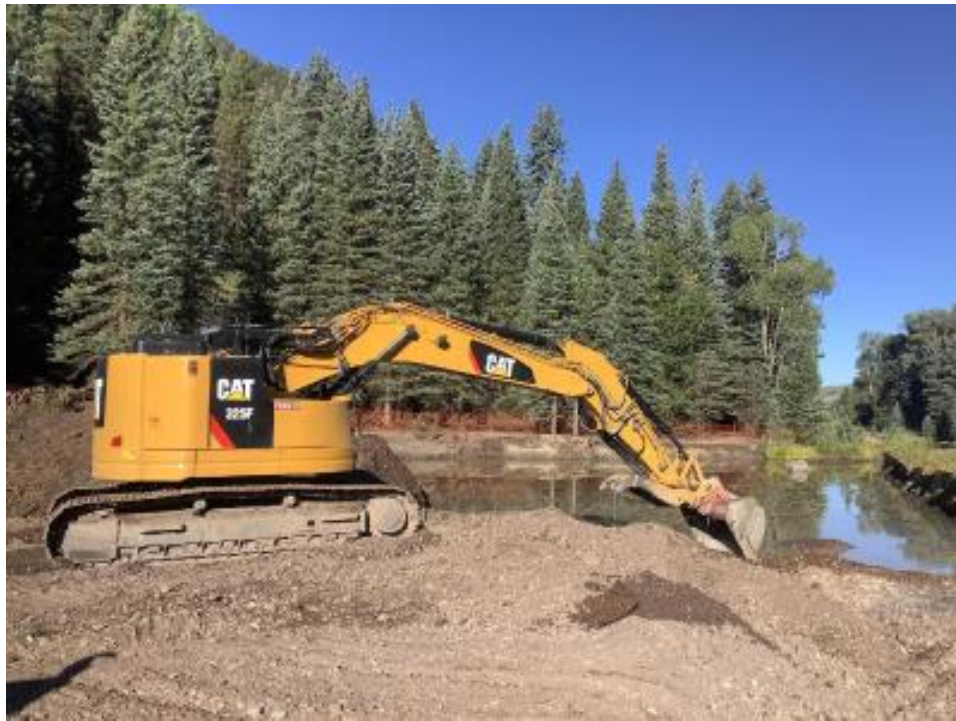
Excavator removes tailings down to water level in western end of ST2.
