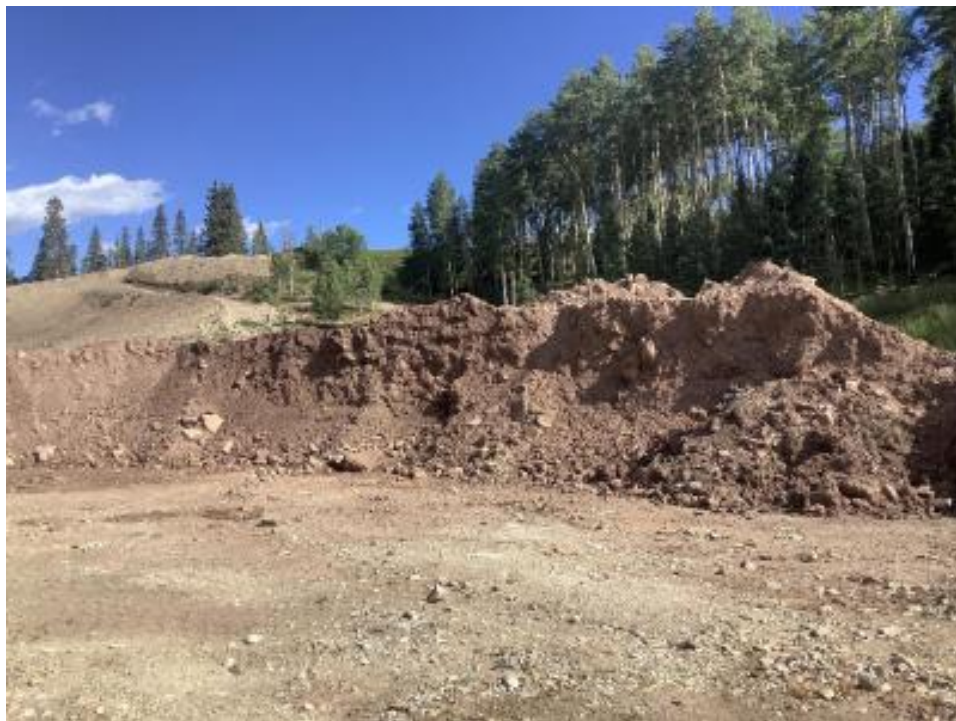
START and EPA screen clean infill dirt provided by San Miguel County for the excavated tailings areas.
