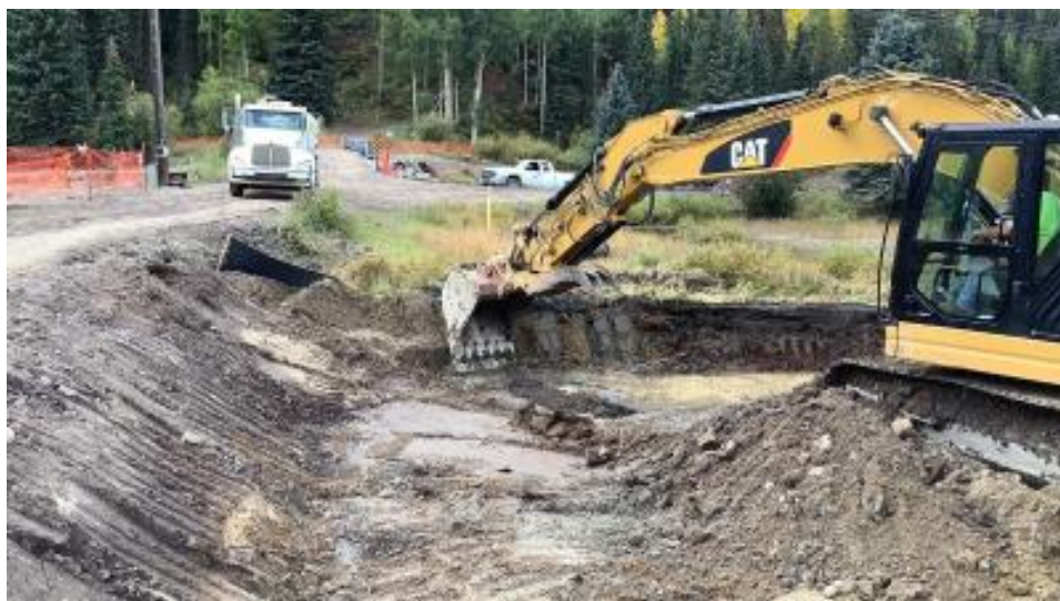
Excavator continues to work in tailings area NTN. Water truck in the background wets down the road to control dust.
