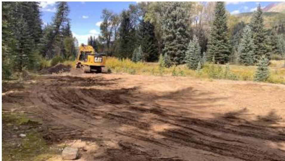
Excavation of mine tailings has begun in area ST3.
