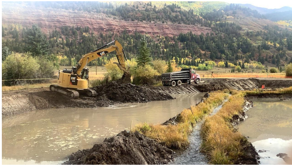
Excavator operator continues to remove mine tailings from NTN, while the fully loaded and tarp covered dump truck prepares to go to the Idarado repository.
