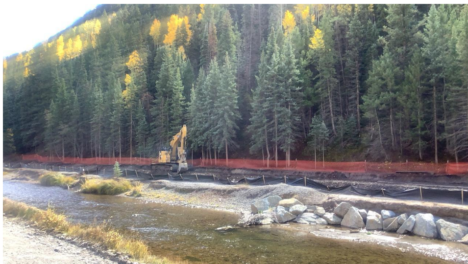
Excavator operator smooths out backfill in ST1 Central in order to create an access road to begin excavation of ST1 South.
