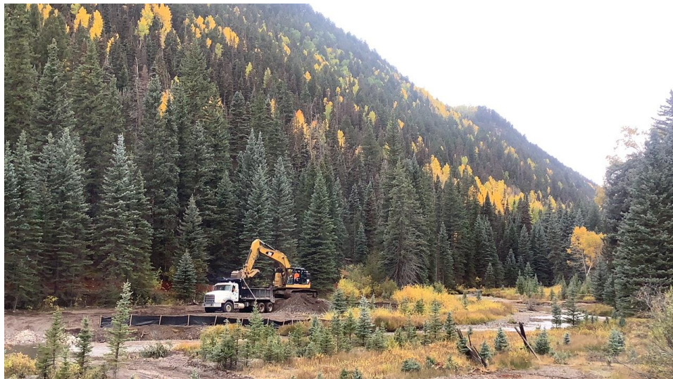
Excavator operator loads a dump truck with mine tailings from area ST3. The tailings will be hauled to the Idarado repository.
