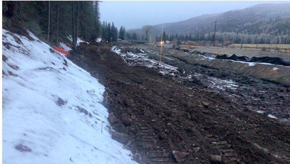
Mine tailings from ST1 South have been fully excavated. The area has also been completely backfilled with clean material.
