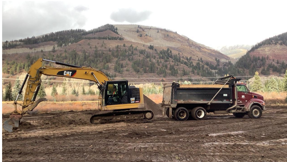
Excavator works in borrow source to load dump truck with clean backfill material.
