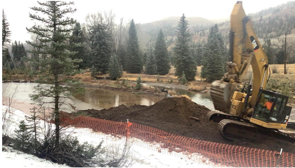
Excavation of ST3 is approximately 90% complete. The operator has piled up the excavated tailings in order to load dump trucks more efficiently.
