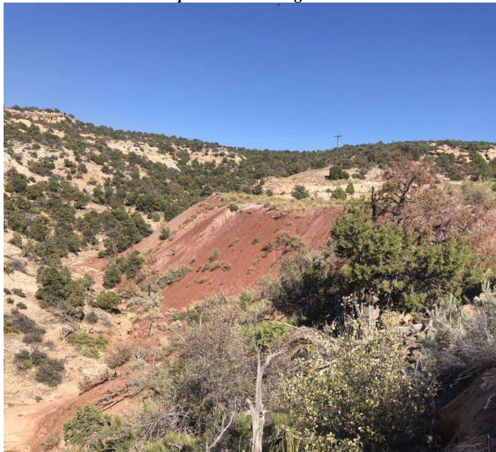
Photo 2: Mine Waste in Ephemeral Drainage at the Radon Mine
