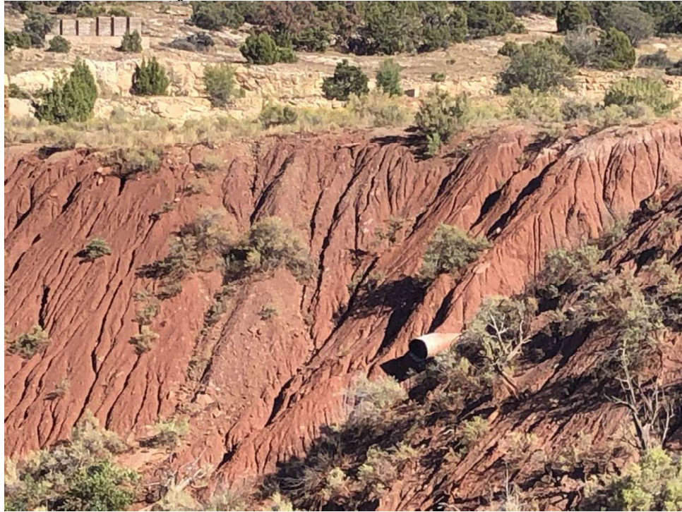
Photo 2: Mine Waste in Ephemeral Drainage at the Radon Mine
