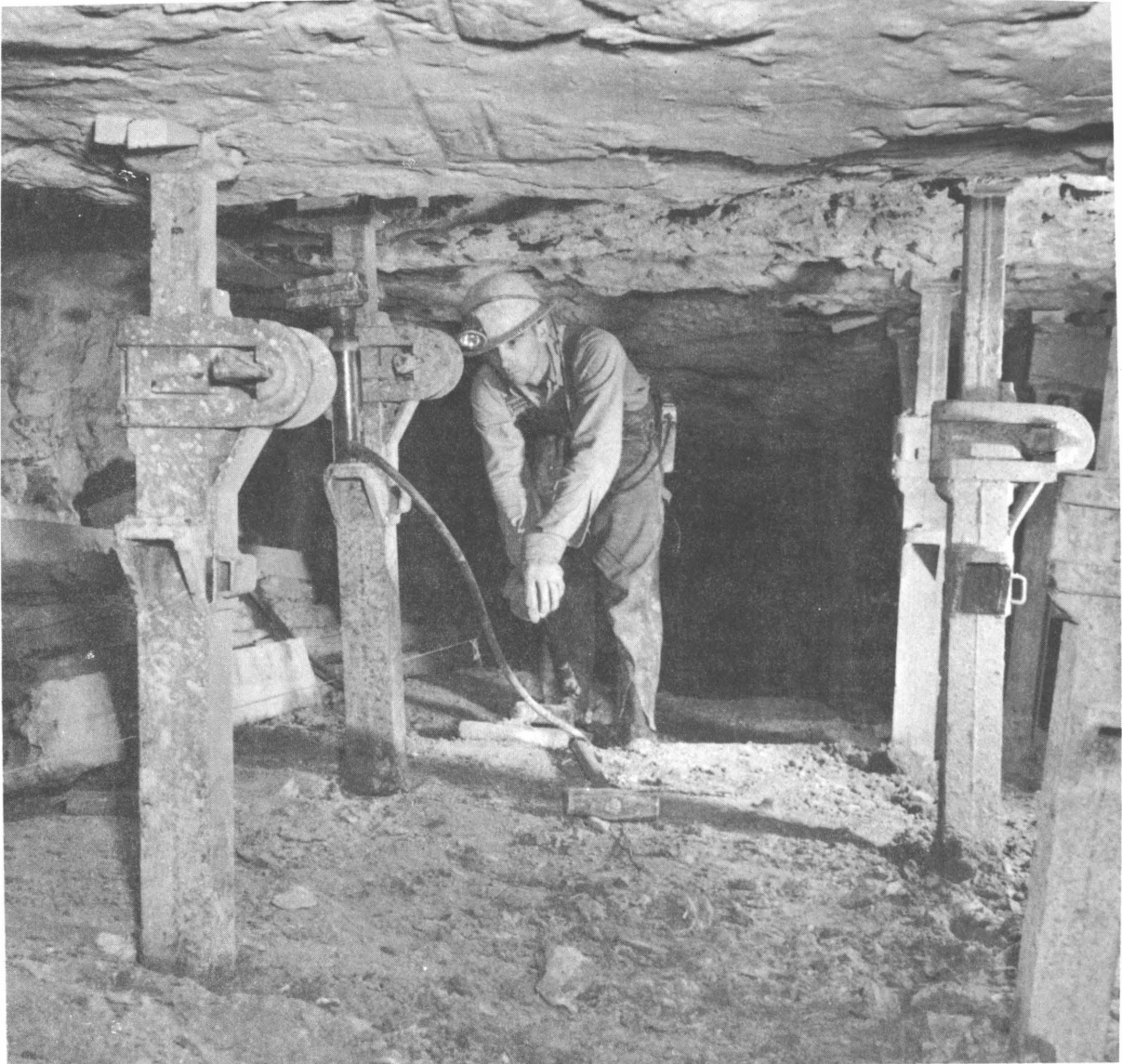
FIGURE 12. - Setting Prop Along New Line.
