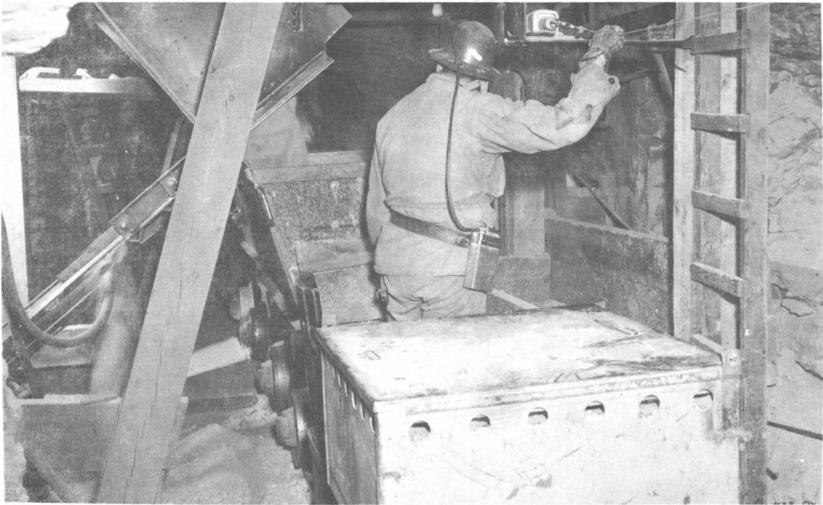
FIGURE 19. - Loading on the Haulage Level.
