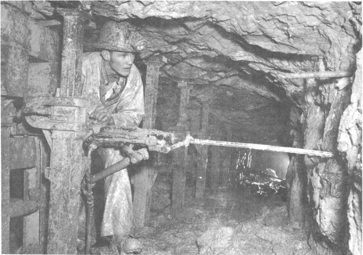
FIGURE 7. - Drilling Wet at Longwall Face.
