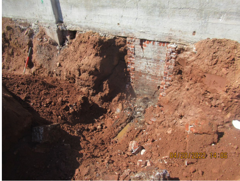
Building A Sewer Disconnection at North Wall – 5/2022 (#17)
