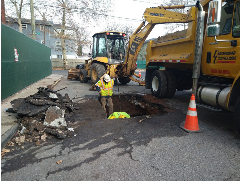
Building A Waterline Disconnection located in 6 th Street – 11/30/2021 (#12)
