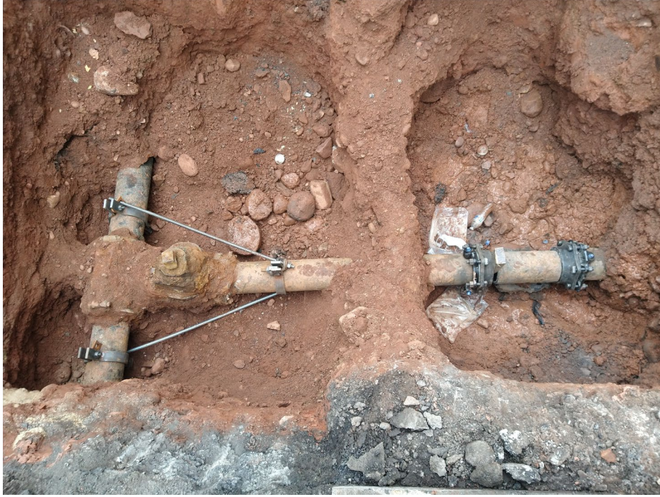
Building B 6-inch Waterline Disconnection at Bergen Street – 11/22/2021 (#7)
