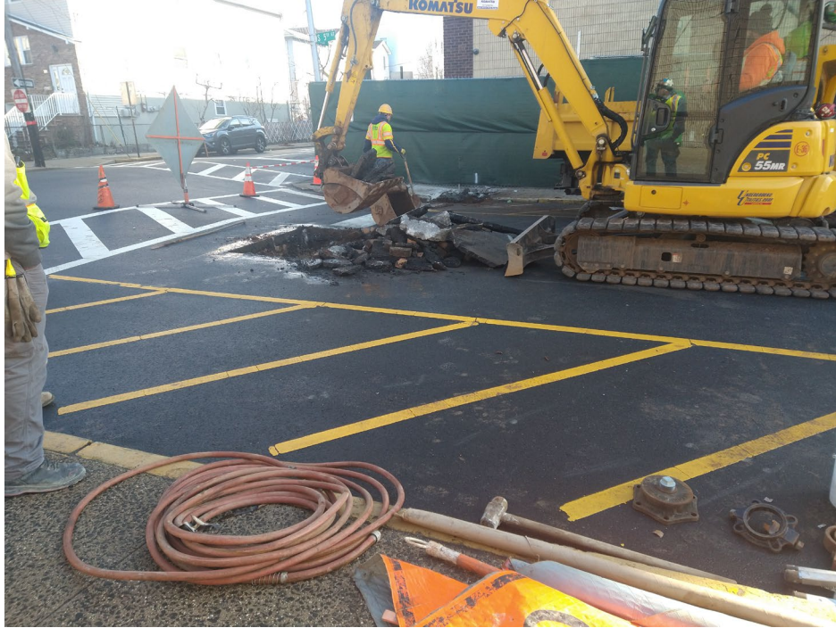
Building A Excavate for 8-inch Waterline Disconnection at Sussex and 5 th – 2/8/2022 (#14)
