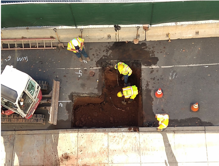
Building B Excavation for Waterline Disconnection at Bergen Street – 11/9/2021 (#7)
