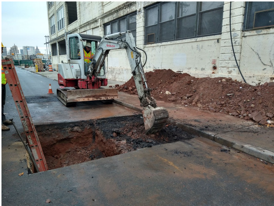
Building B Preparation to Disconnect 6-inch Waterline on Bergen Street – 11/22/2021 (#7)
