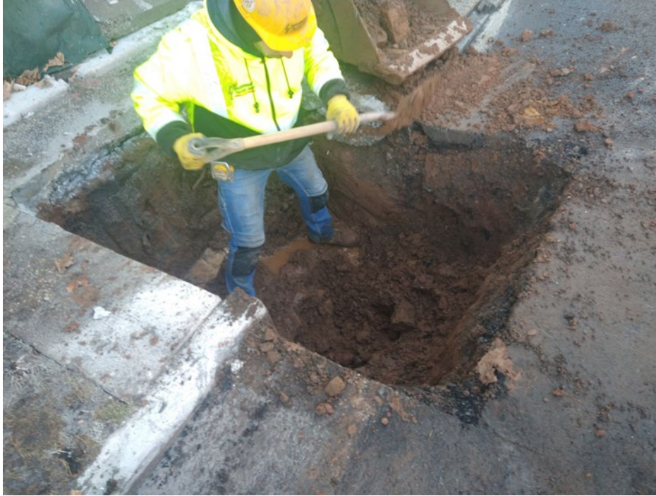
Building A – Excavate for 6-inch Waterline Disconnection – 2/8/2022 (#13)
