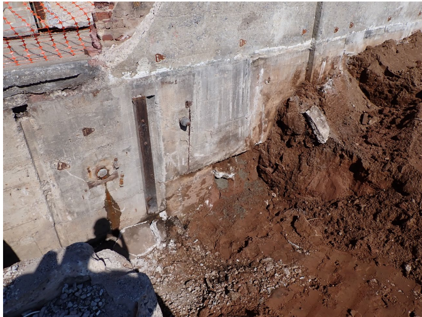
Building A Sewer Disconnection at West Wall – 5/2022 (#17)
