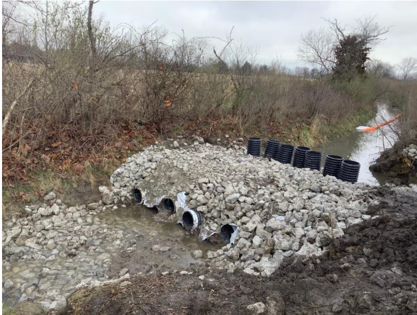
Underflow dam installed at Erie Road.
