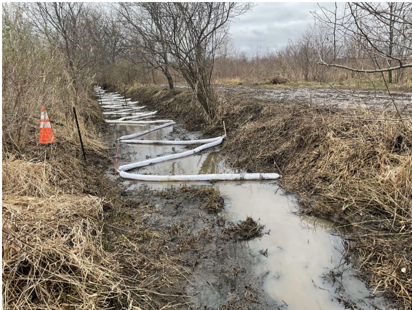
Boom placed between Sunoco and US-23 along North Tenmile Creek.
