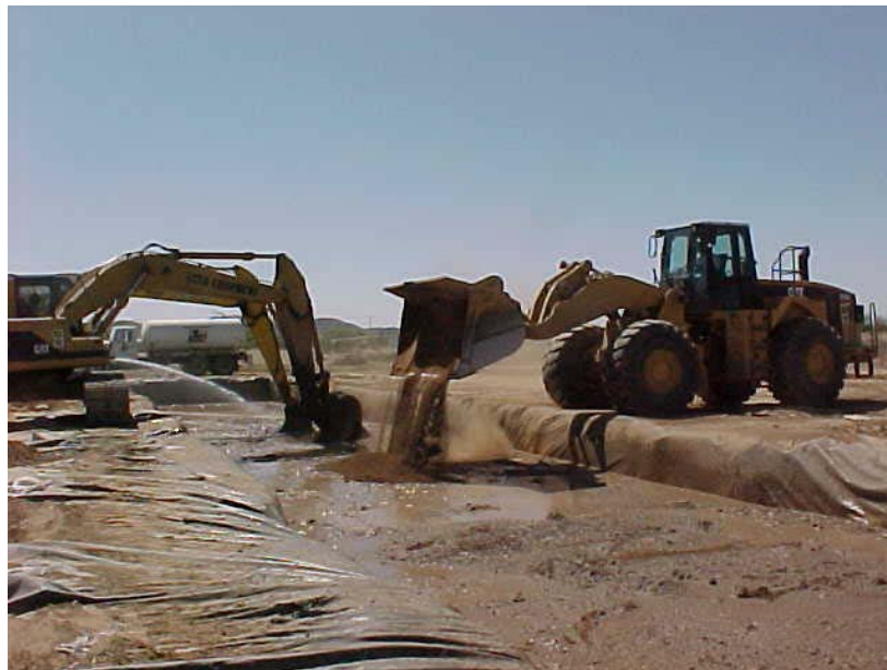
Photo 6: Addition of soil, nutrients, and water to treatment cell.
