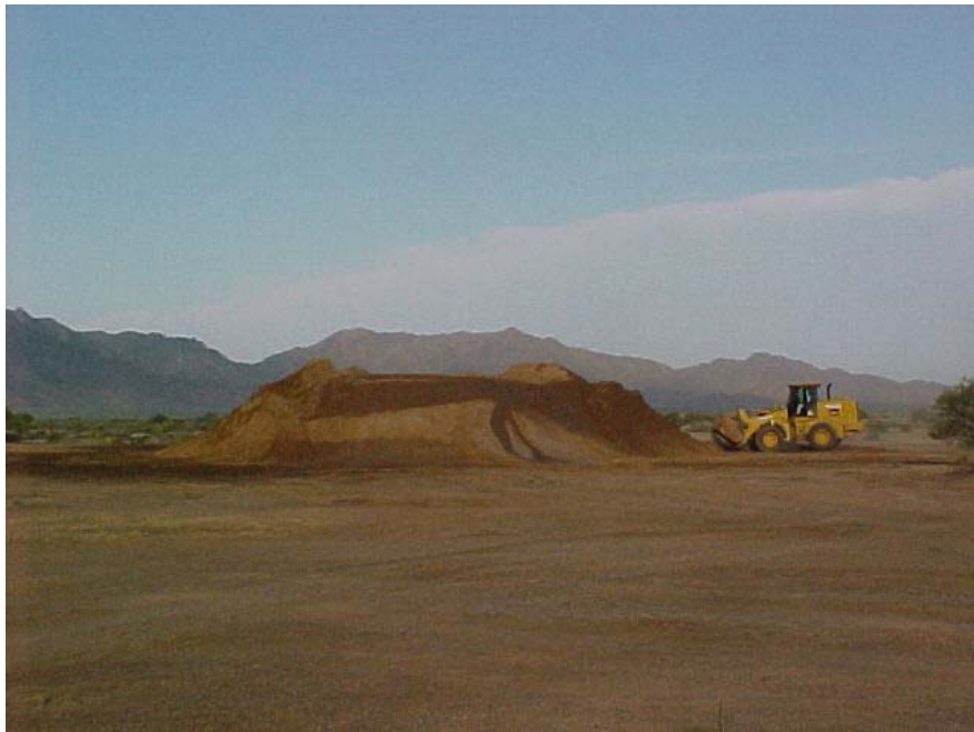
Photo 3: Stockpile of toxaphene-contaminated soil awaiting treatment.
