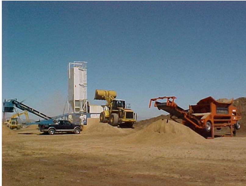
Photo 5: Treatment cell construction: pugmill and sieve in operation.
